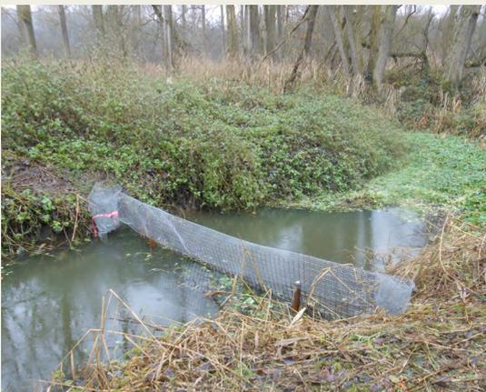
Fig 124. In order to prevent the spread of fragments, a containment net was placed in the stream. Photo: Province du Brabant Wallon
