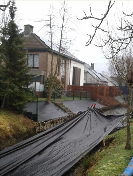
Fig 111. Geotextile light-blocking covers were placed in order to compress vegetation and exclude sunlight during a few years. Photo: Provincie Oost-Vlaanderen dienst Integraal Waterbeleid
