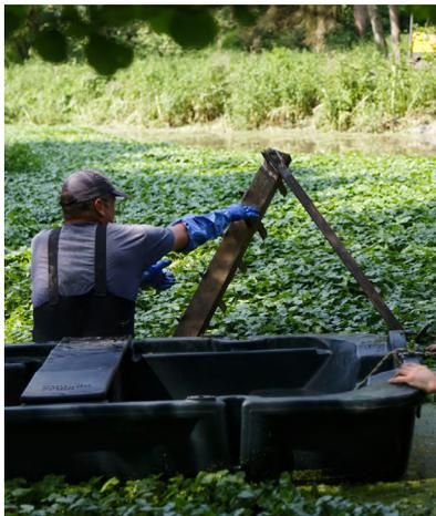
Fig 20. Large rake being pulled by a winch from the bank helping operators to remove important quantity of plant material. Photo: Adrien Latli
