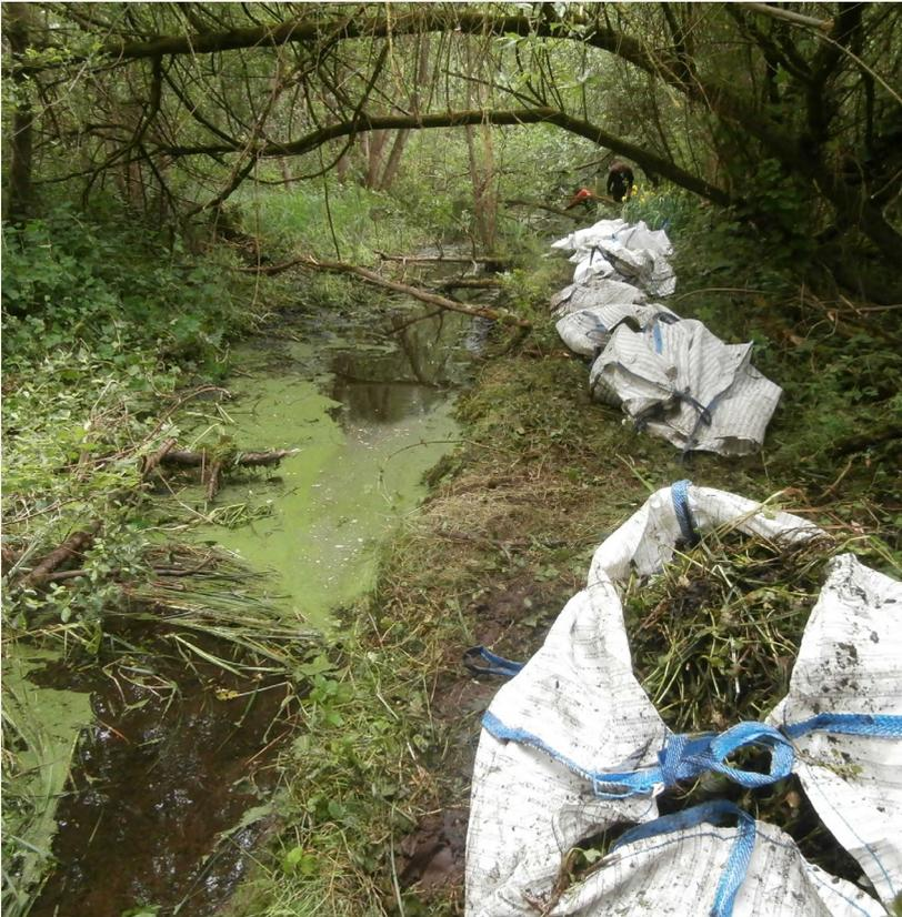
Fig 126. The harvested plant material was stored in flex containers before being exported to a refuse depot. Photo: Province du Brabant Wallon
