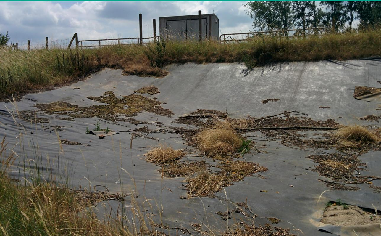
Fig 102. It is necessary to check for any damages that would allow the plant to grow through the sheeting. Photo: Marijke Thoonen
