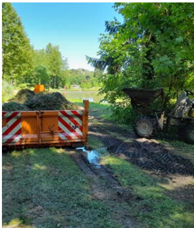
Fig 5. Small dumper truck used to transport the harvested plant material to the container. Photo: Dido Gosse
