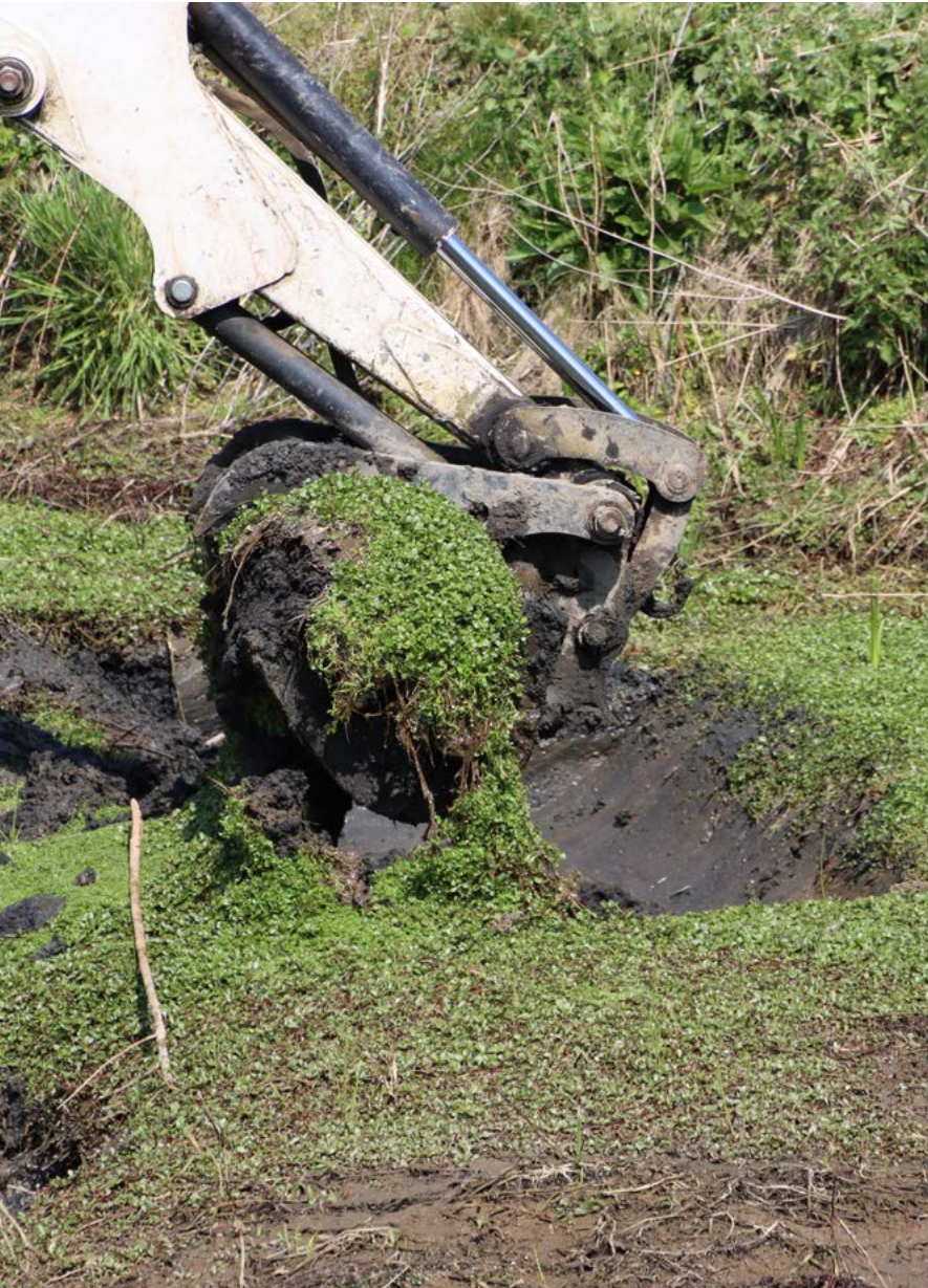
Fig 9. Mechanical dredging of water primrose after a complete drainage of the water body. Photo: Arnaud Monty
